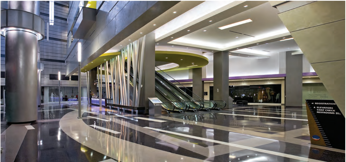
The multi-layered atrium of the World Market Center in Las Vegas features an extensive labyrinth of coves. Thousands of linear feet of eW ® Cove Powercore, an LED cove fixture from Philips Color Kinetics, provide seamless blending of light in runs of up to 50 feet. Color consistency from fixture to fixture and across individual fixtures' beam spread (color spatial uniformity) is especially important in high-profile, angle-dependent lighting installations such as this one.
