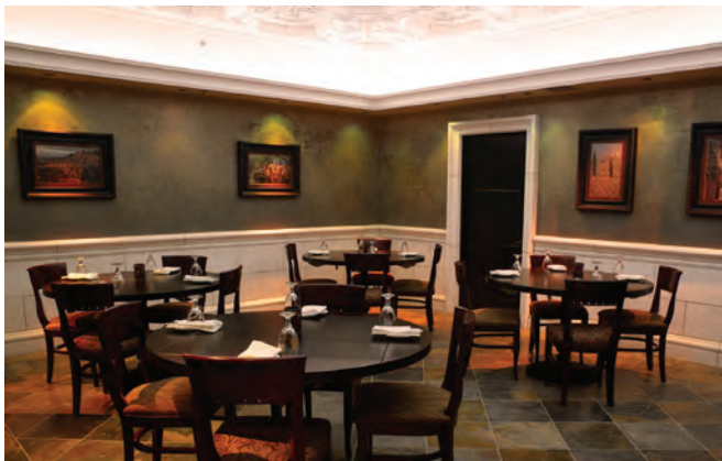
iW® Cove Powercore, tunable white-light LED fixtures with channels of warm and cool LEDs, allow the staff of Boston's Rustic Kitchen to dial in the exact shade of white light they desire — cooler for daytime (above), warmer for night (below).
